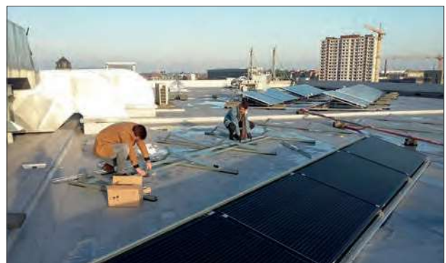
Installing the solar panels on the roof.
